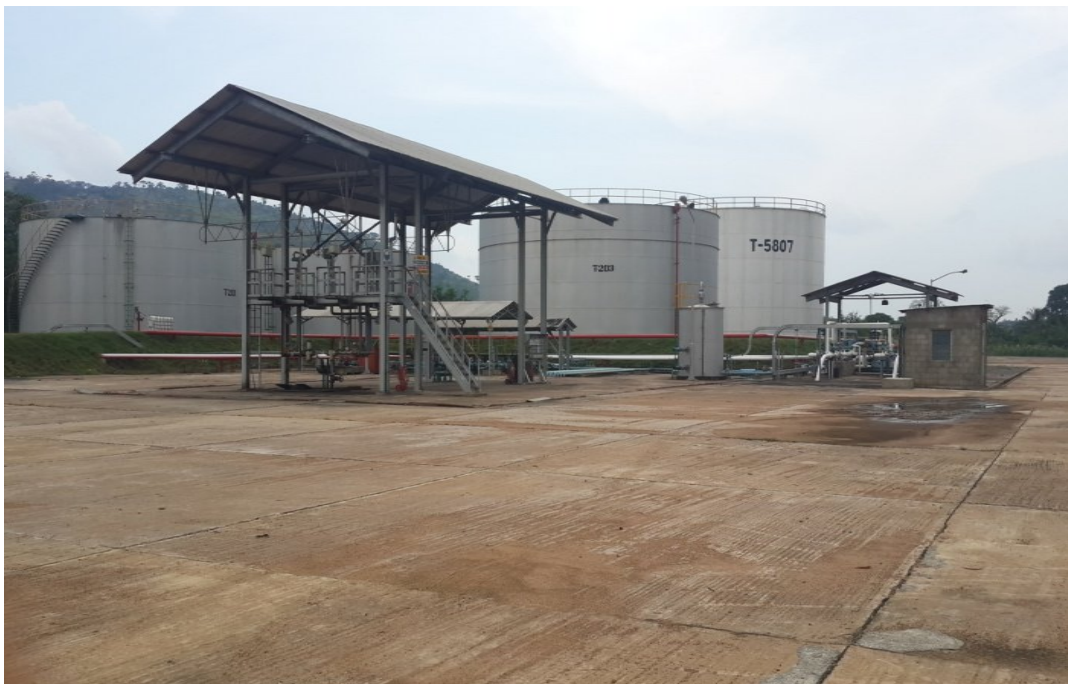
Source: Audit Team Date Taken: 08/11/2013
